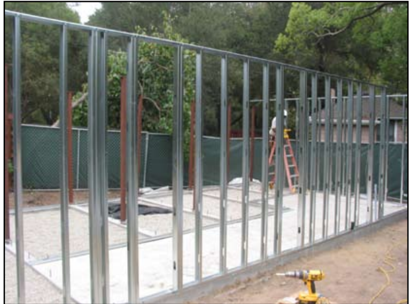
Aviary floor and wall framing.
