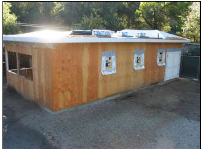
Progress continues on the aviary at the Santa Barbara Museum of Natural History. Photo by John O’Brien
