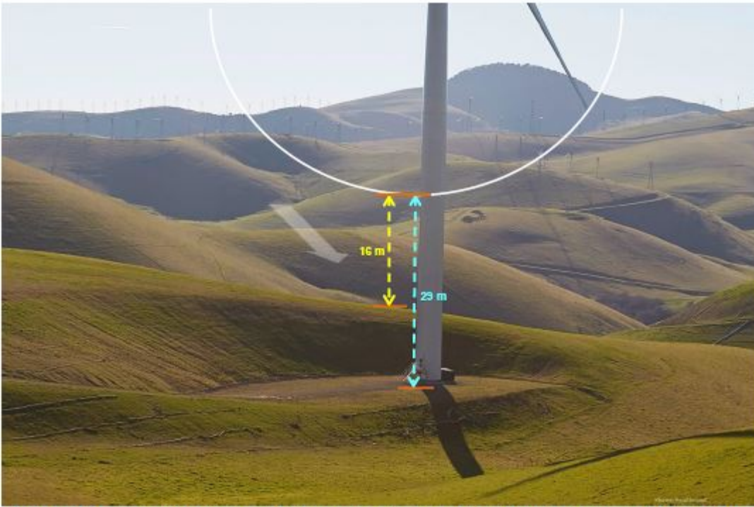
Figure 14. This view is toward the prevailing wind (see broad white arrow), so the prevailing upwind slope, the crest of which is only 30 m from the wind turbine, forces any bird or bat passing over it into a vertical gap of only 16 m between the hill crest and the low reach of the blade. The wind turbine's dimension of 29 m height above ground of the low reach of the rotor has lost its meaning due to the effects of grading of a pocket into the slope. I have seen this type of grading across the western USA.
