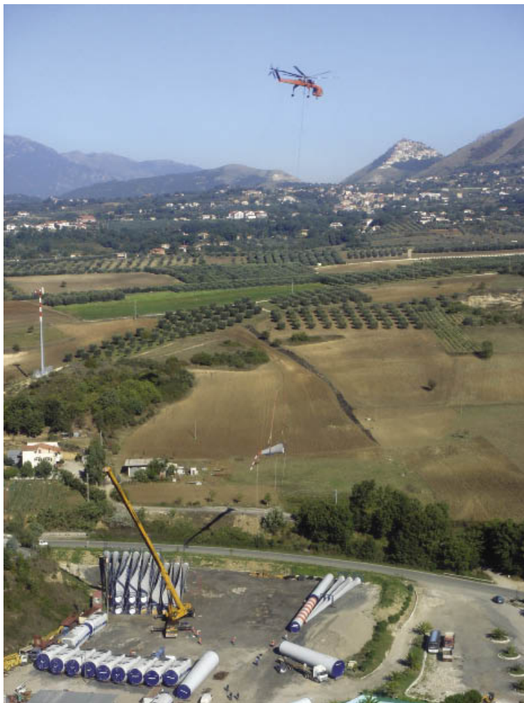
Transport of WTG blades by heavy-lift helicopter
